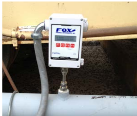
The Model FT2A - shown here reading fuel to a burner used in aggregate drying for asphalt production - is being used as a part of a company-wide efficiency improvement program by a FOX customer operating multiple locations across the U.S..
