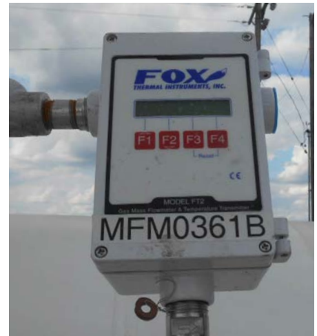
Shown here installed in a fuel line to a furnace, the Model FT2A flowmeter and temperature transmitter is ideal for use in a great variety of industrial and harsh environment applications.
